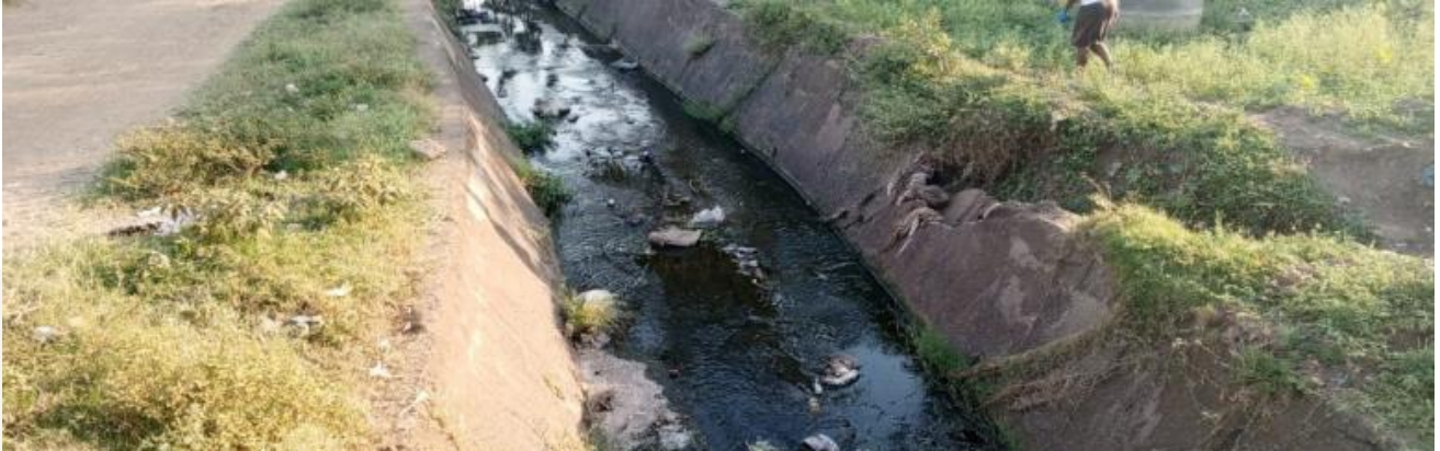
Figure 28: Image of blocked drainage facility
